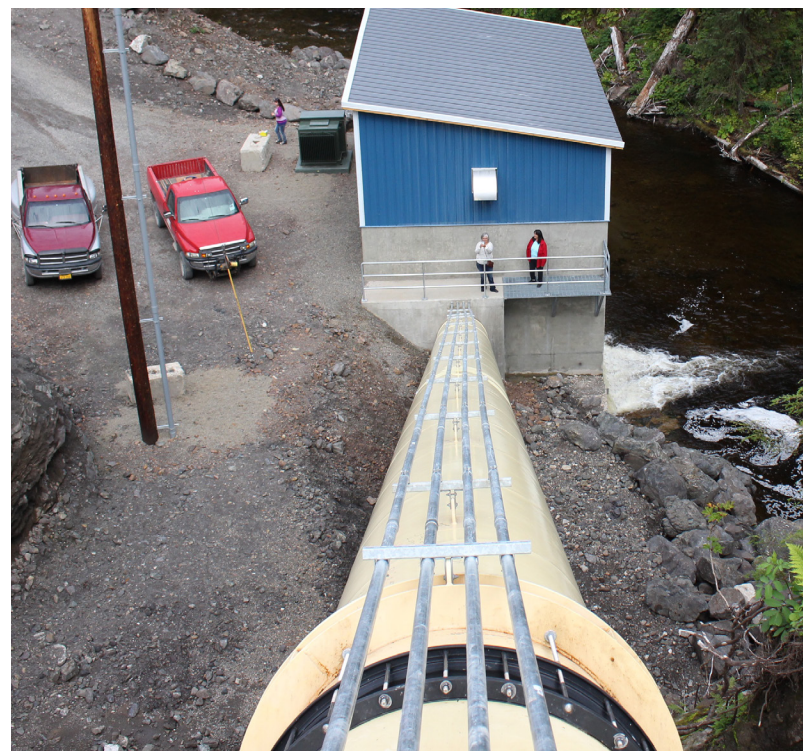
Water flows down the tube and spins a turbine that creates electricity. (Photo by Elizabeth Jenkins, courtesy of KT00)
